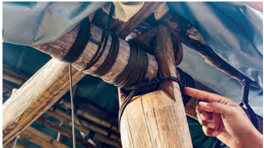
Expert hale builder Nalani Tukuafu demonstrates the system of notching and lashing used in the construction of traditional hale structures, which are held together only with lashing. In this image, a traditional hale currently under construction at Kaunani in Keaukaha, Hilo, is protected from the elements with a tarp before thatching.
