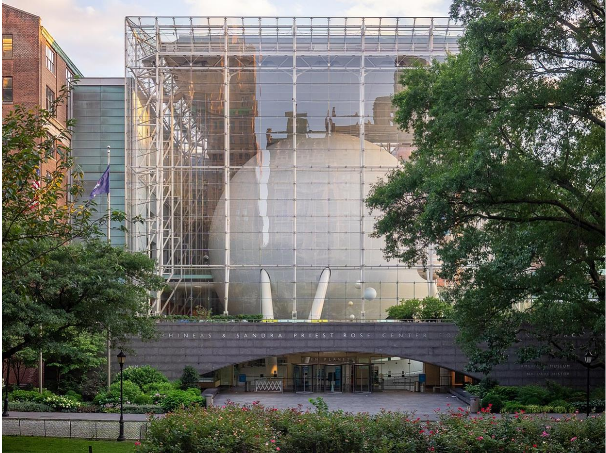
Figure 7. American Museum of Natural History, Rose Center for Earth and Space, New York City, NY, 2000. Project Architect: Kalavati Somvanshi. Firm: Ennead Architects.
