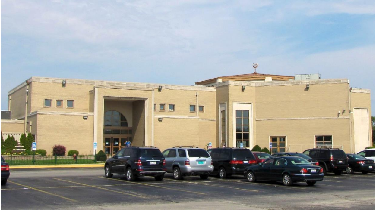
Figure 5. Islamic Foundation Mosque, Villa Park, IL, 1990s. Architect: Khatija Asif Ali Hashmy.
