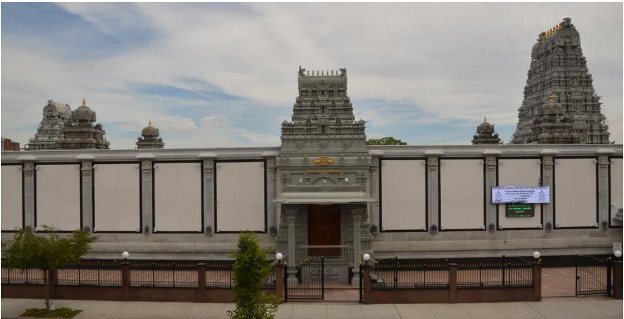
Figure 2. The Hindu Temple Society of North America, also known as Ganesh Temple, Flushing, Queens, NY, 1977. Architect: Barun Kumar Basu
